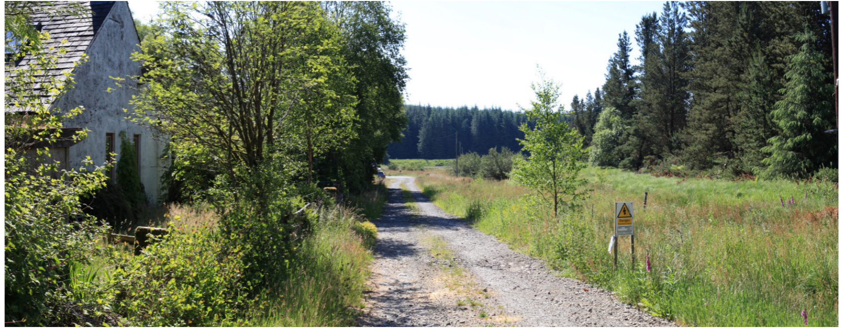
South-western elevation and access track. Ground floor bedroom windows.
