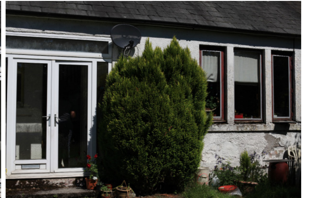
South-eastern elevation. Main entrance and living/dining room.
