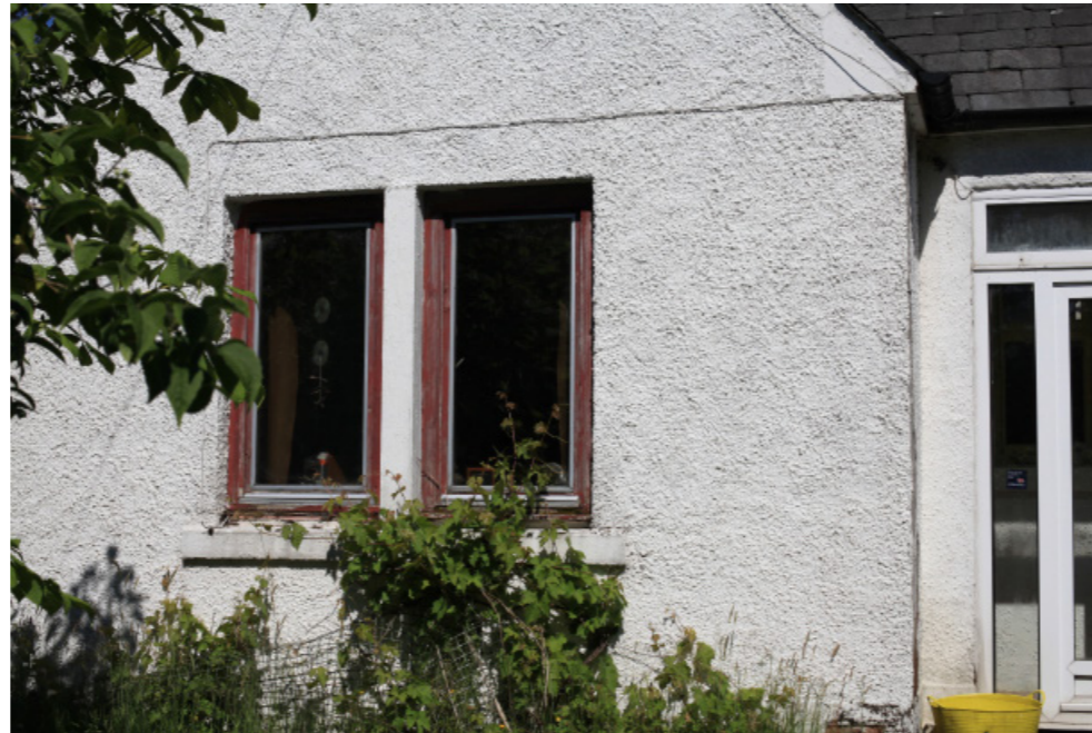
South-eastern elevation. Ground floor bedroom windows.
