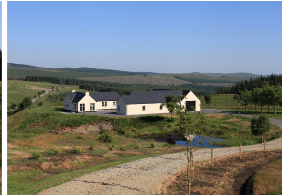
Second house to the south of the main house. View of the western elevations of house and out buildings.
