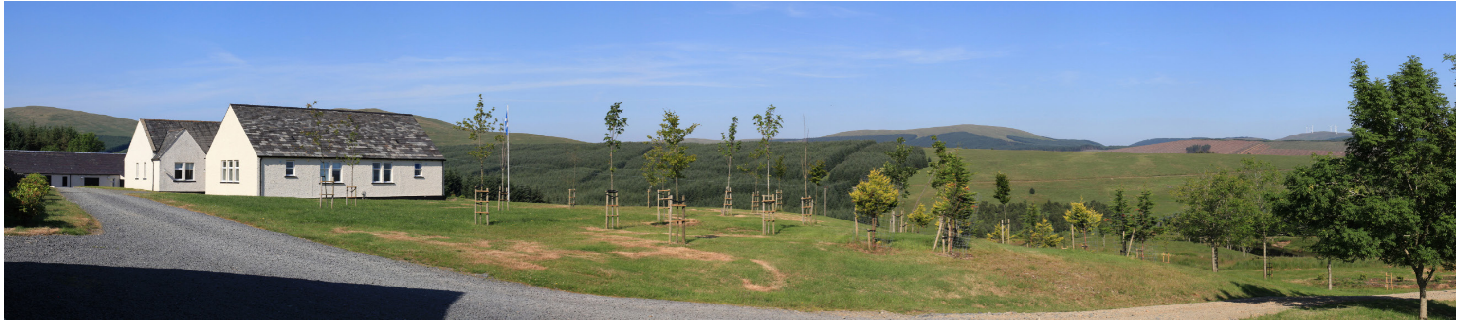
View north-east from PROW to the south of the main house showing new building/extension to the southern side of the house.
